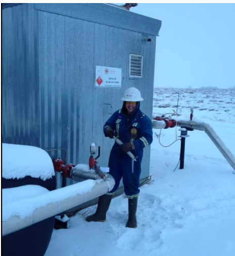
Orifice plate and chart change for gas well volume measurement (Evan):
